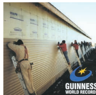
Workers installing the longest piece of stainless steel siding.
